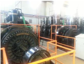
2 of the Original 1936 Fairbanks- Morse Engines
