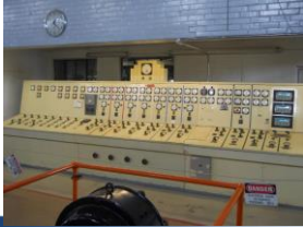
Original Control Panel
