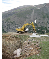
Setting pre-cast Shaft Panels
