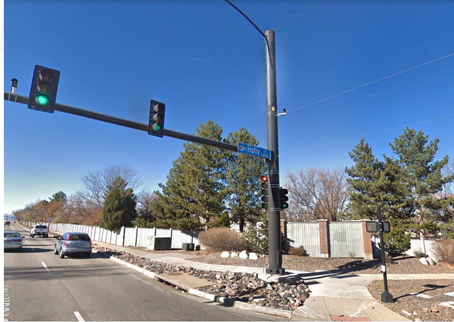
Concealed Equipment Enclosure
