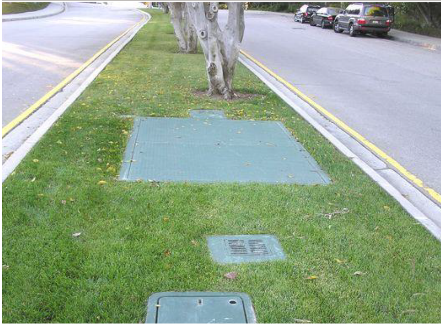
Underground Communication Vault
